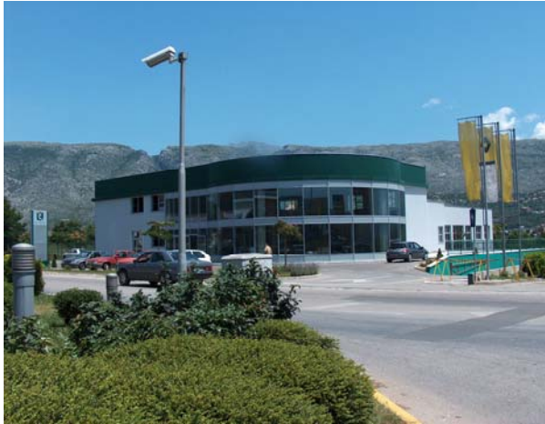
West part of new IGH-MOSTAR LLC building
